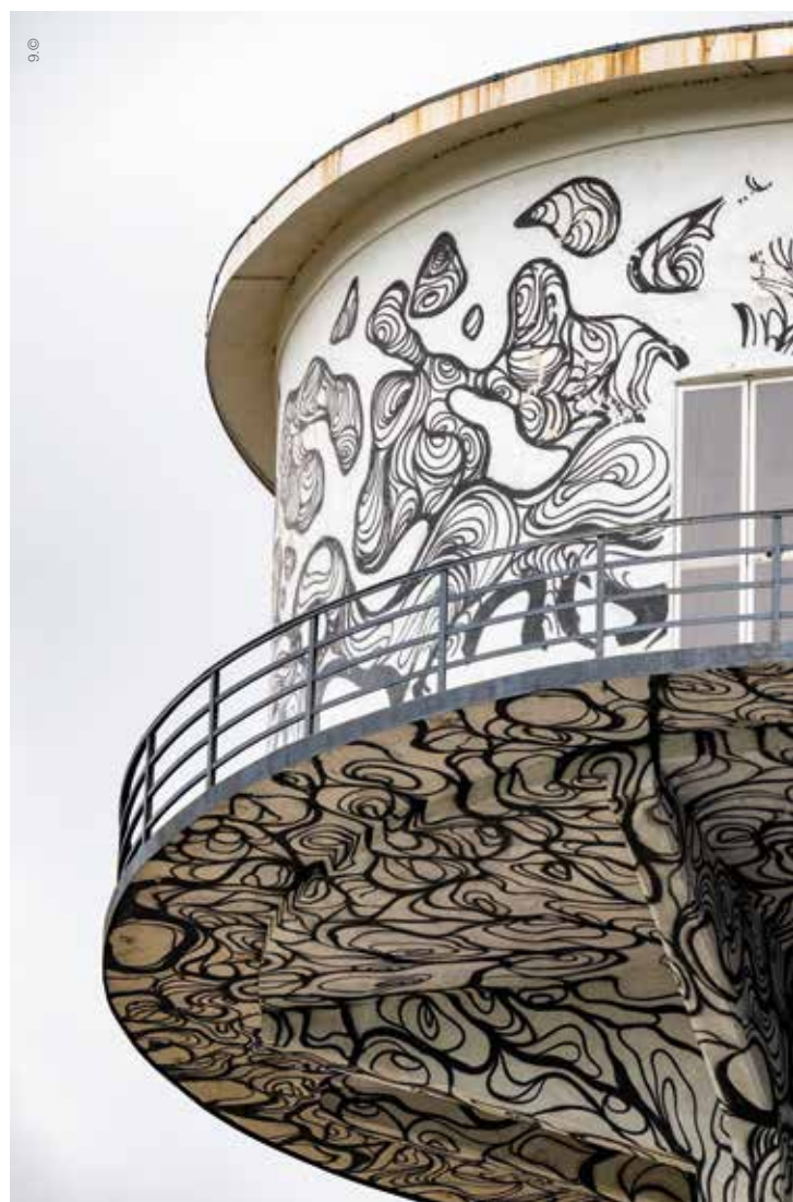
The water tower, a NOI Techpark icon
